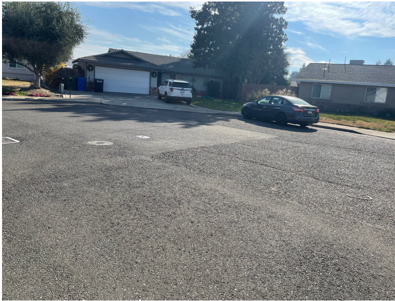
Photo 2: Torrey Court (Patched and Not Patched Portions)
