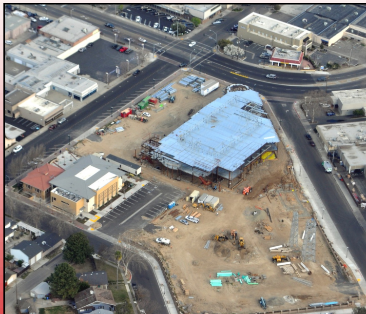
Aerial view of the Public Safety Facility under construction
